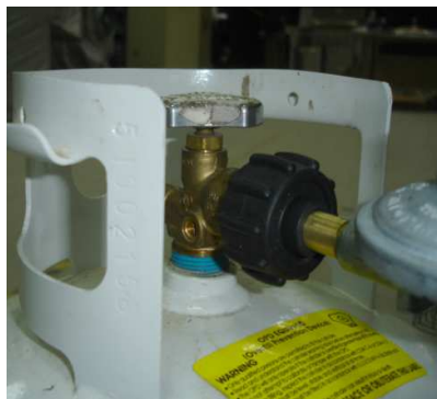
Regulator connects to the gas tank.
